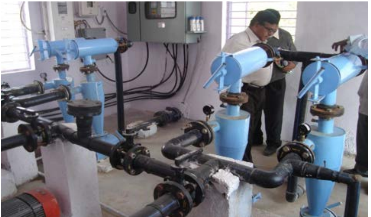
Figure3.9. Inspection of PINS by the officials
