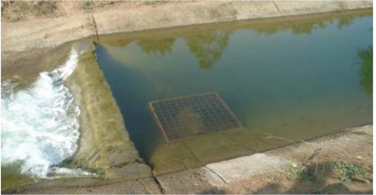
Figure 3.6: Inlet Arrangement for Canal PINS
