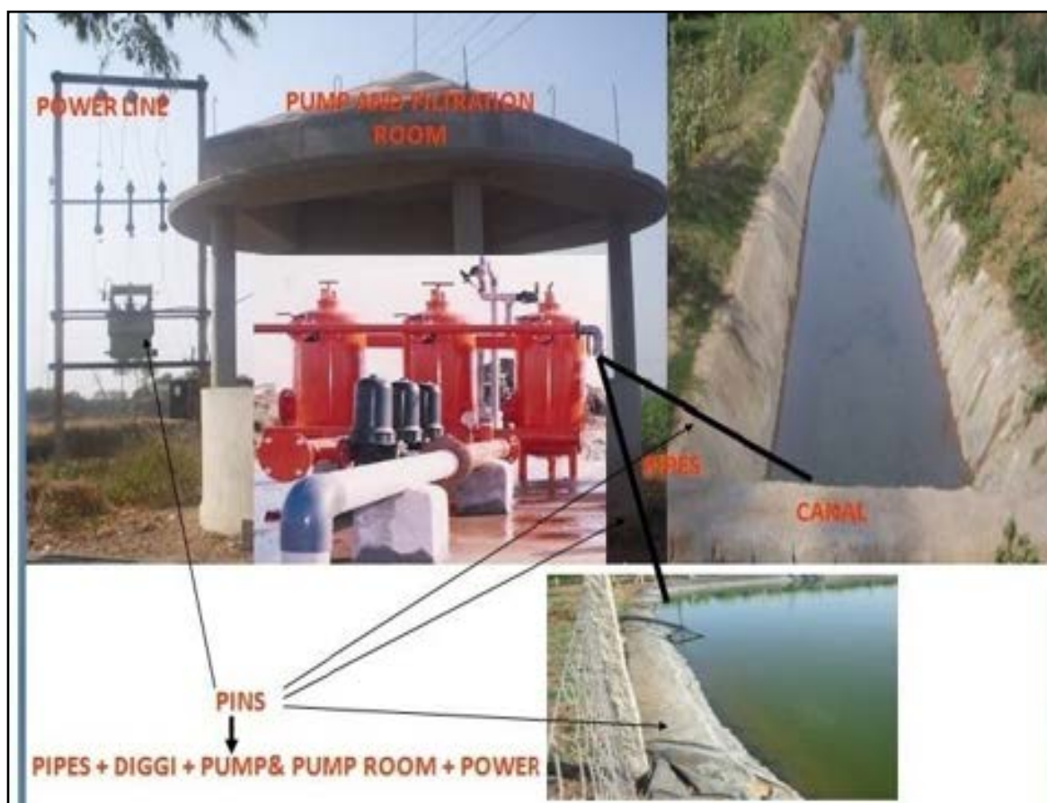
Figure 1.2: Components of PINS in Gujarat
