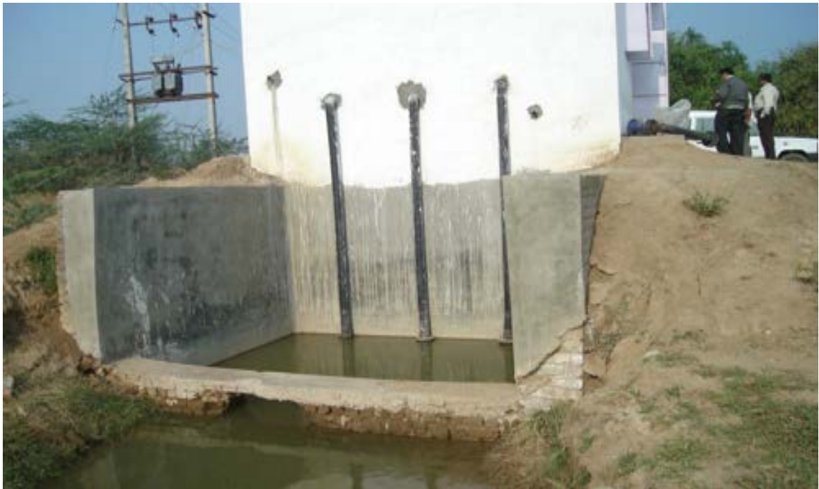
Figure 3.7: Intake Arrangement through Tank
