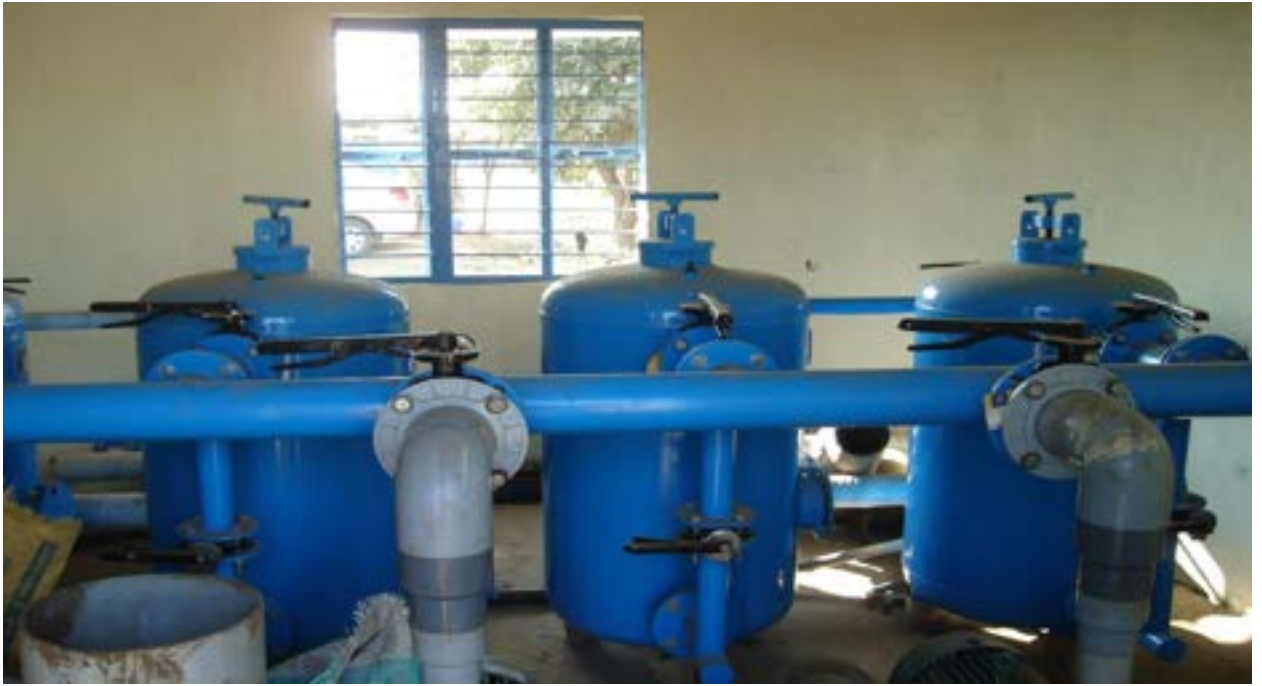
Figure3.8: Inside Arrangements and Filtration units for PINS
