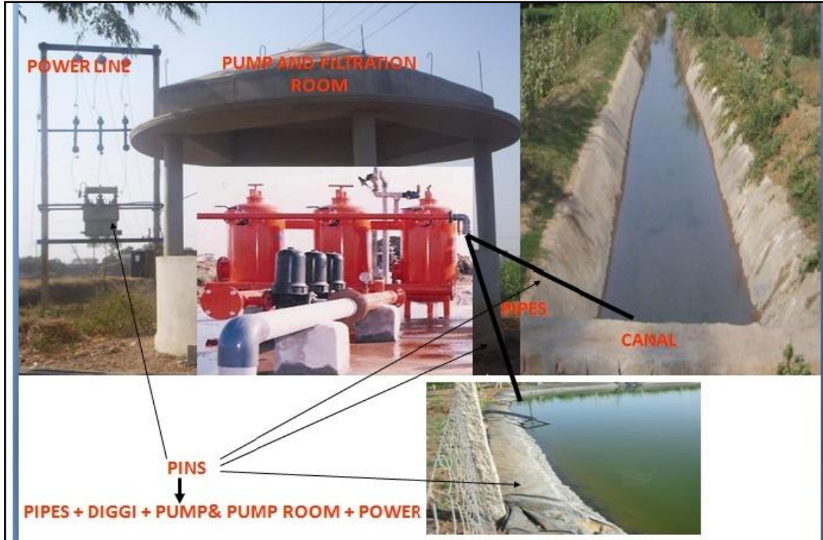
Figure 1.2. Components of PINS
