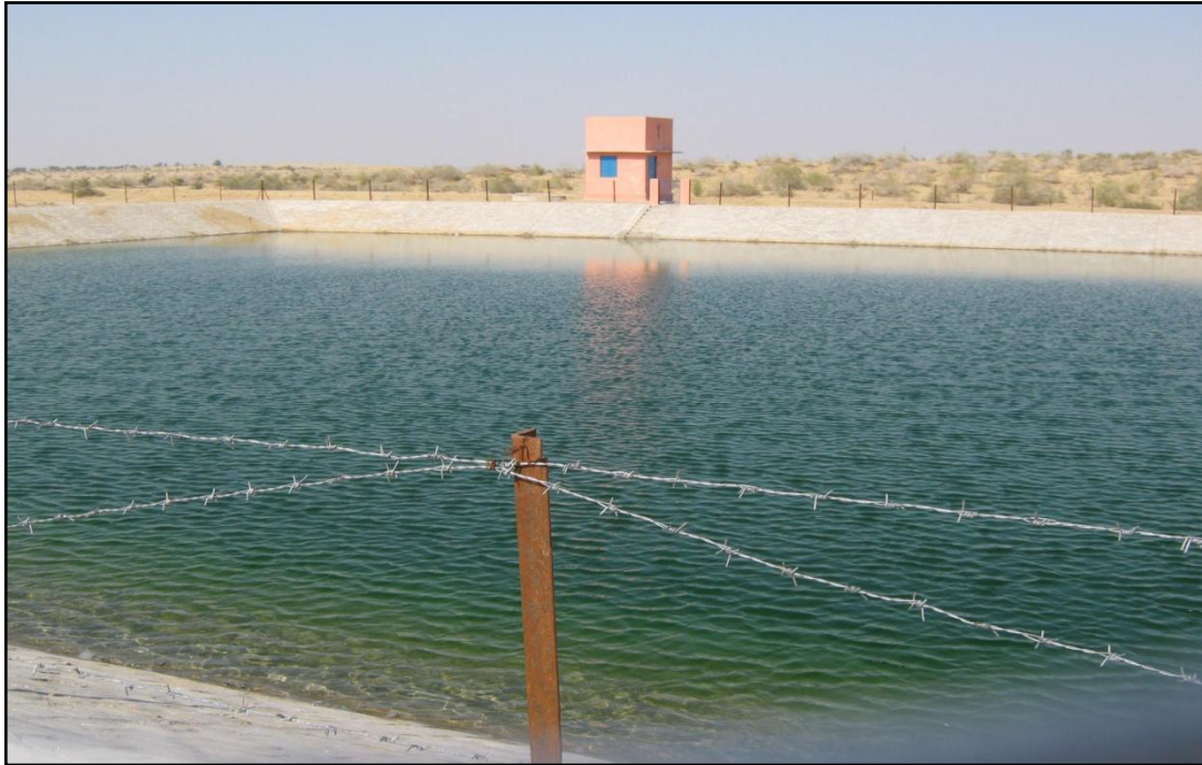
Figure 3.2 Diggi for storage of water in Rajasthan
