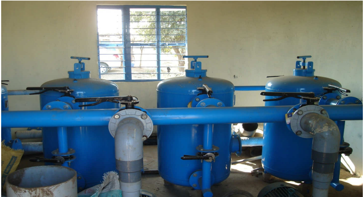
Figure3.8: Inside Arrangements and Filtration units for PINS
