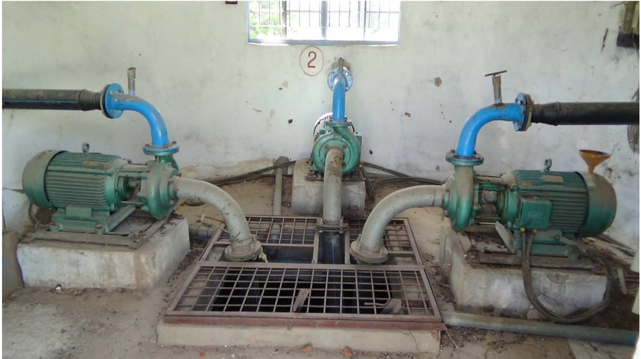
Figure 5.7: Dysfunctional pump sets inside the pump house due to non-utilization
