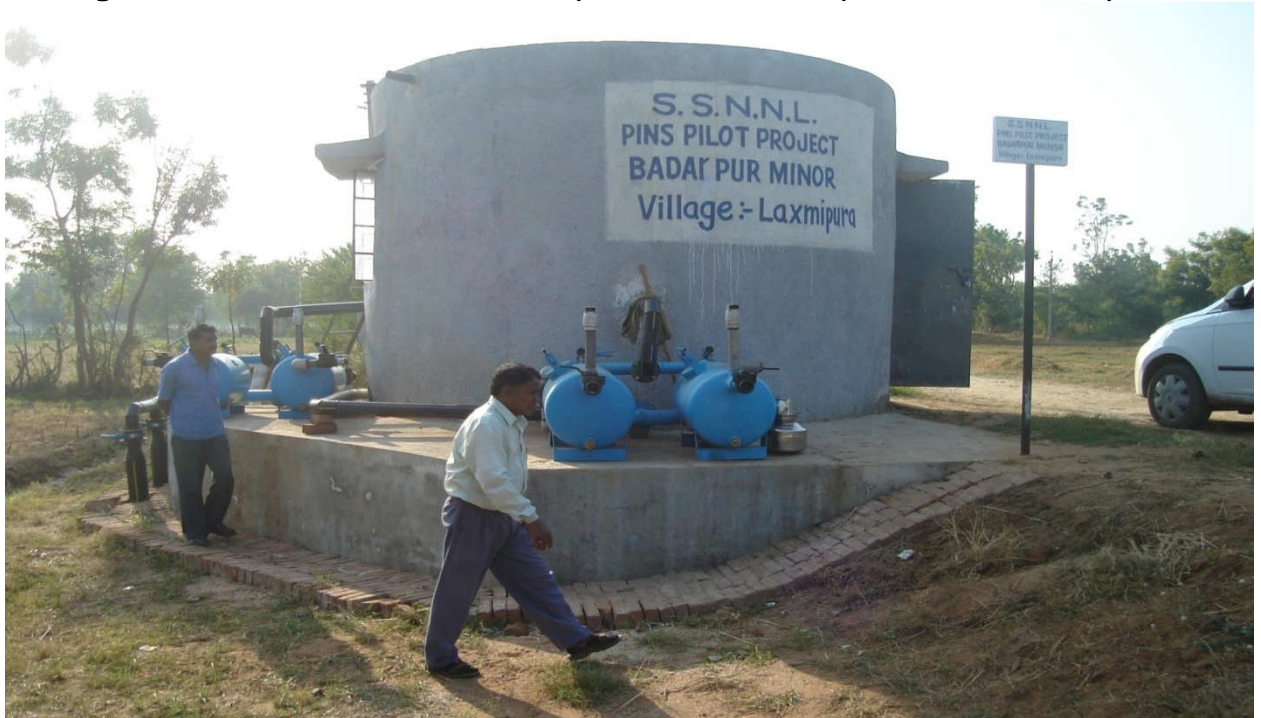
Figure 3.4: Intake Well Cum Pump House at Badarpur Minor, Laxmipura
