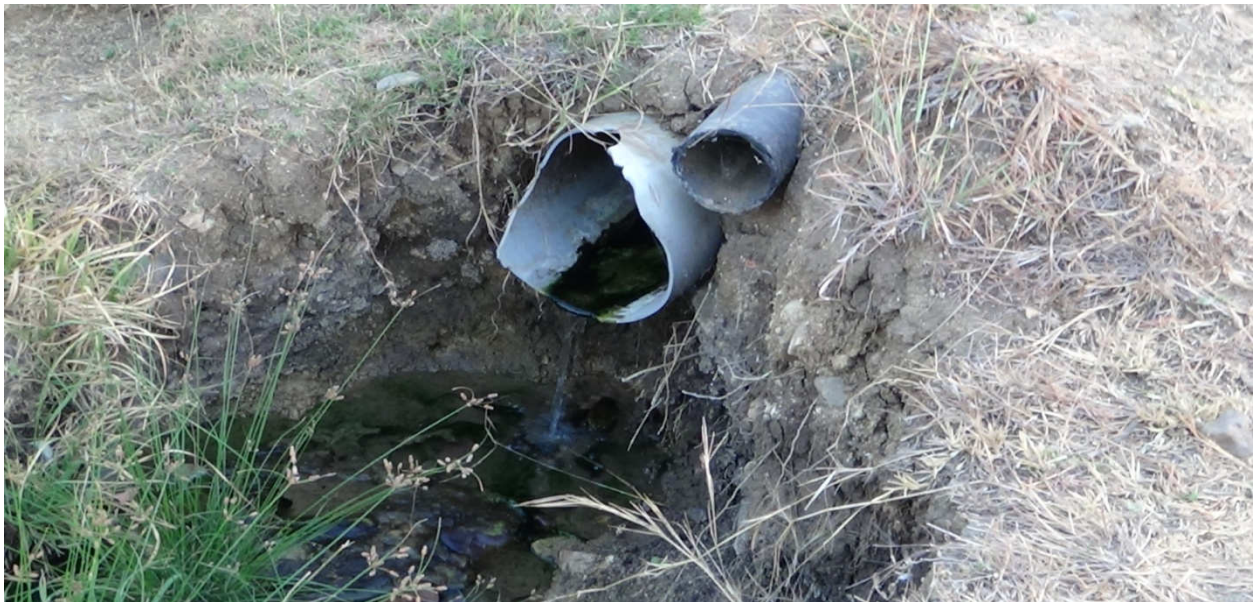
Figure 5.8: Damaged Pipelines upto farmers field from PINS
