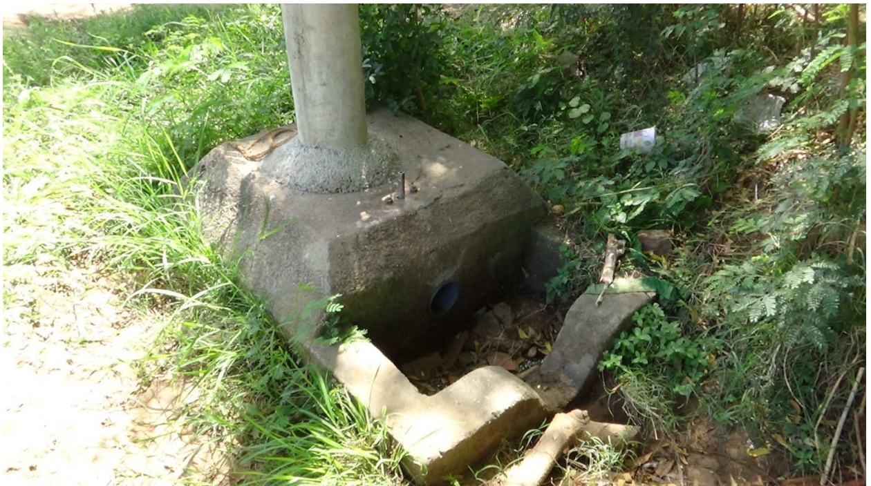
Figure 5.13: UGPL Outlet provided at Farmer's field
