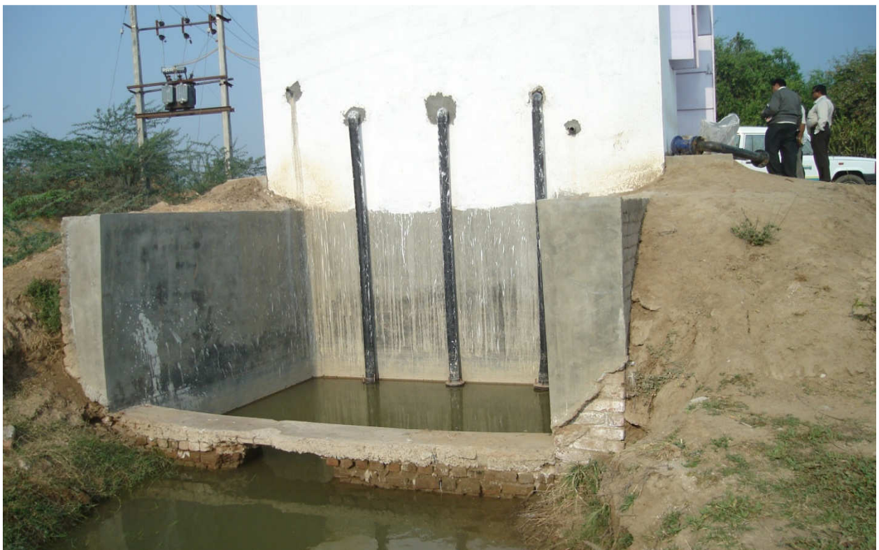
Figure 3.7: Intake Arrangement through Tank
