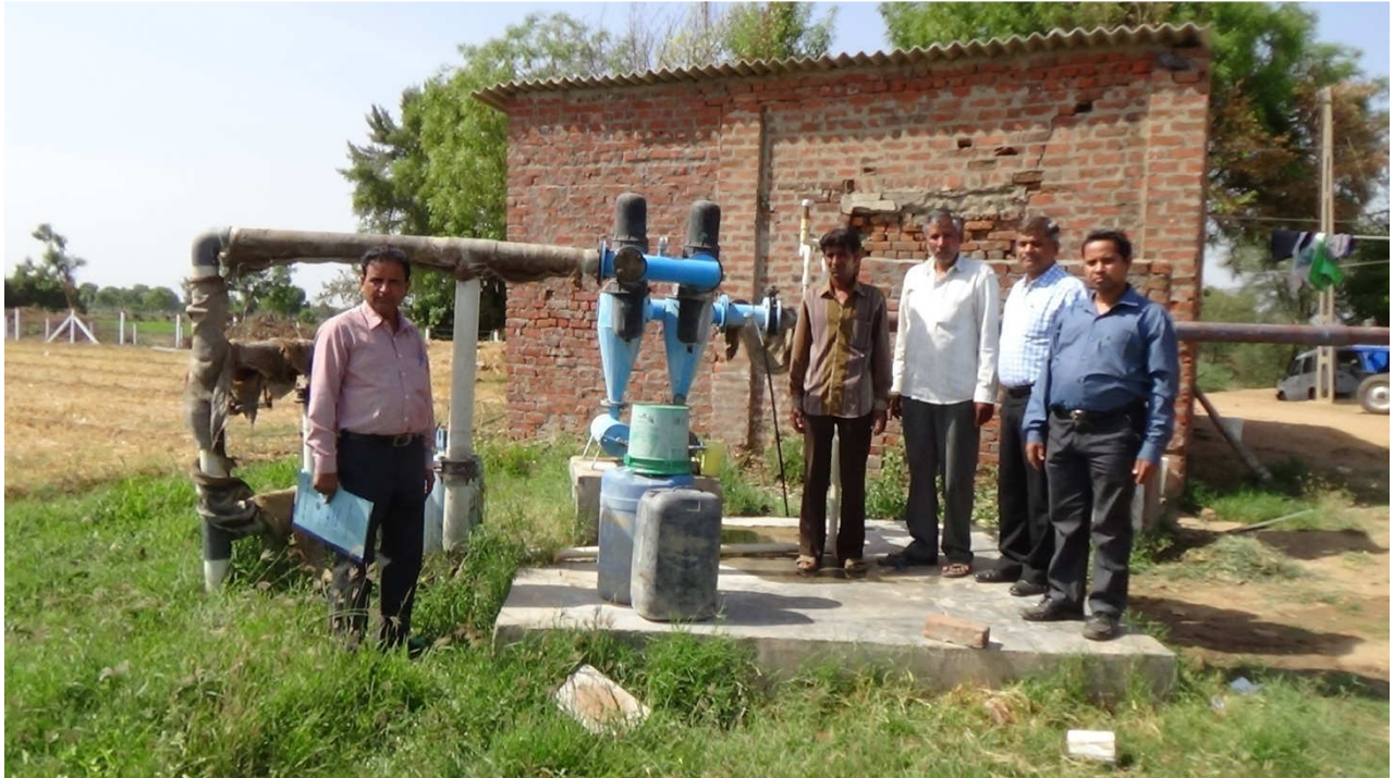
Figure 2.12: Tubewell PINS in Gandhinagar district, Gujarat
