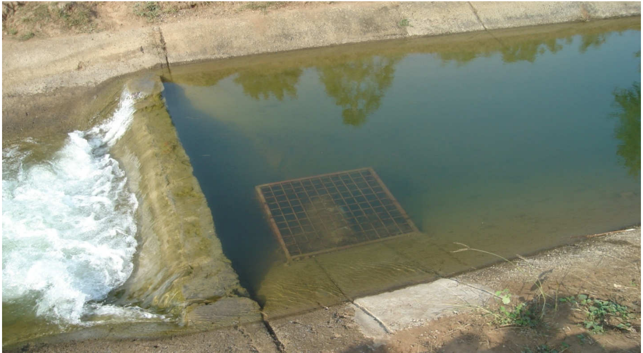
Figure 3.6: Inlet Arrangement for Canal PINS
