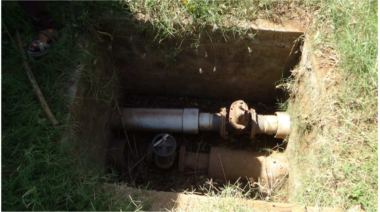
Figure 5.12: Regulating Valve to manage supply of UGPL water to certain plots
