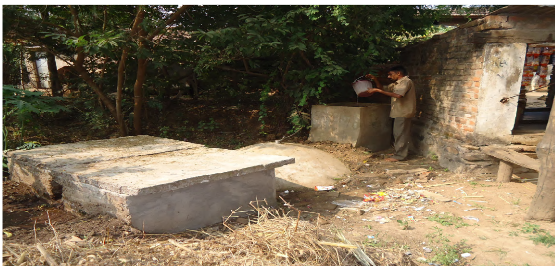
Figure 3.13 Biogas plant at village Simal Faliya of Chhota Udepur
