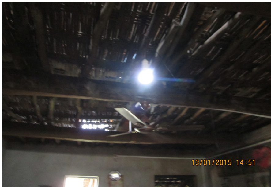
Figure 3.12. Solar Home Light System (HLS) being used by rural households
